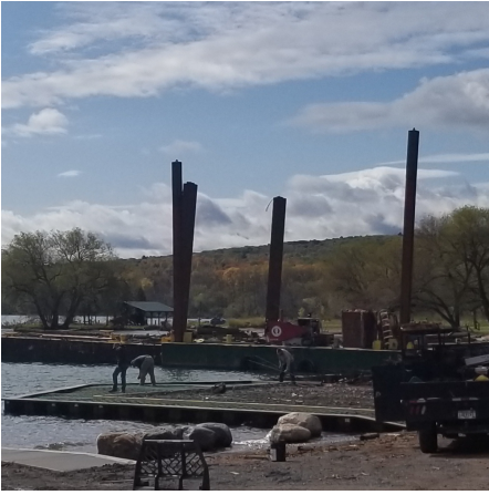
Work in progress at West End boat launch and shoreline.
