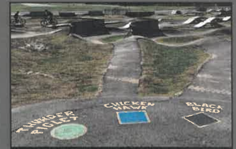
SLOPESTYLE ZONE - ASPHALT SURFACING
