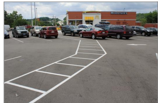
Exhibit 17-1. A pedestrian crosswalk in the parking lot of a fast food restaurant
