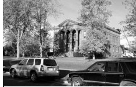
Bayfield County Courthouse (SWB, Inc.)
