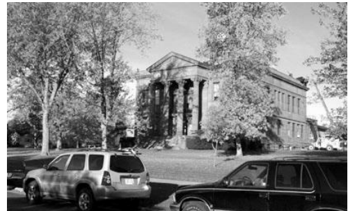
Bayfield County Courthouse (SWB, Inc.)
