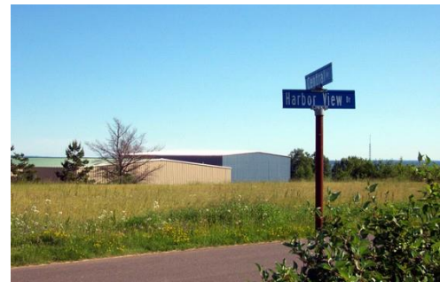
View from Harbor View Drive of the Back of the Boat Storage Buildings with a Glimpse of the Lake in the Background (SWB, Inc.)
