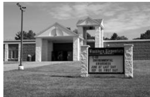
Washburn Elementary School (SWB, Inc.)
