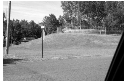
Water Reservoir on Washington Avenue south of Hillside (SWB, Inc.)
