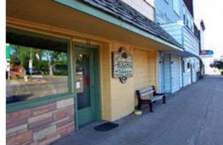
Bayfield Street Commercial Uses (SWB, Inc.)
