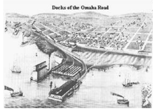
Waterfront and Railroad in the Late 1800s (City of Washburn)
