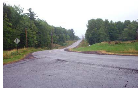
County Road C – Major Collector Road (SWB, Inc.)
