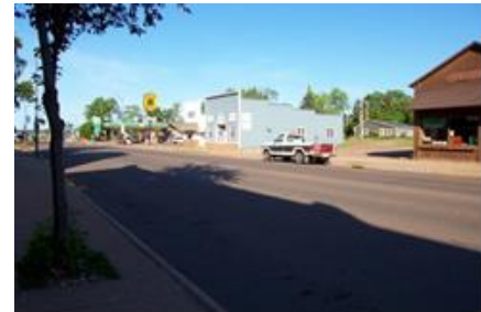
Typical Infill Development Opportunity on Bayfield Street (SWB, Inc.)
