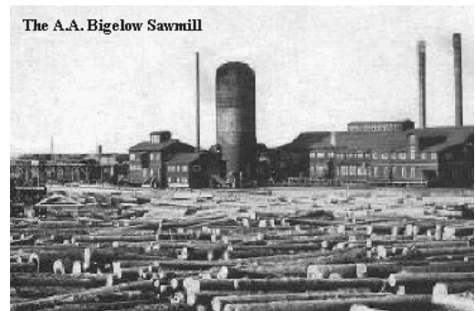
Former A.A. Bigelow Sawmill at 6 th Avenue West (City of Washburn)
