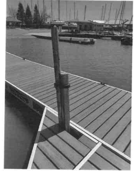
5 S2.0 EXISTING 45° CORNER W/ SLOTTED POCKET
