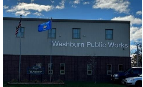
Washburn Public Works (NWRPC)
