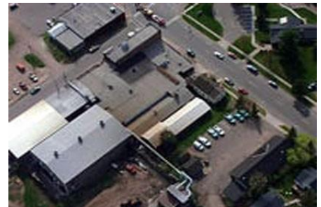
Aerial View of Washburn Iron Works at 112 East Bayfield Street (Washburn Iron Works Website)
