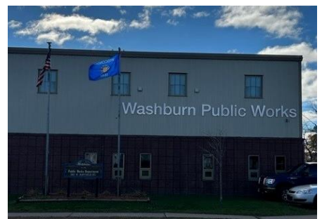
Washburn Public Works (NWRPC)
