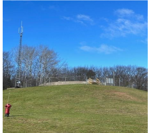
Water Reservoir on Washington Avenue South of Hillside (NWRPC)
