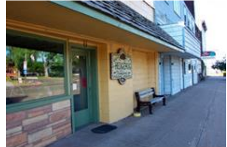
Bayfield Street Commercial Uses (SWB, Inc.)
