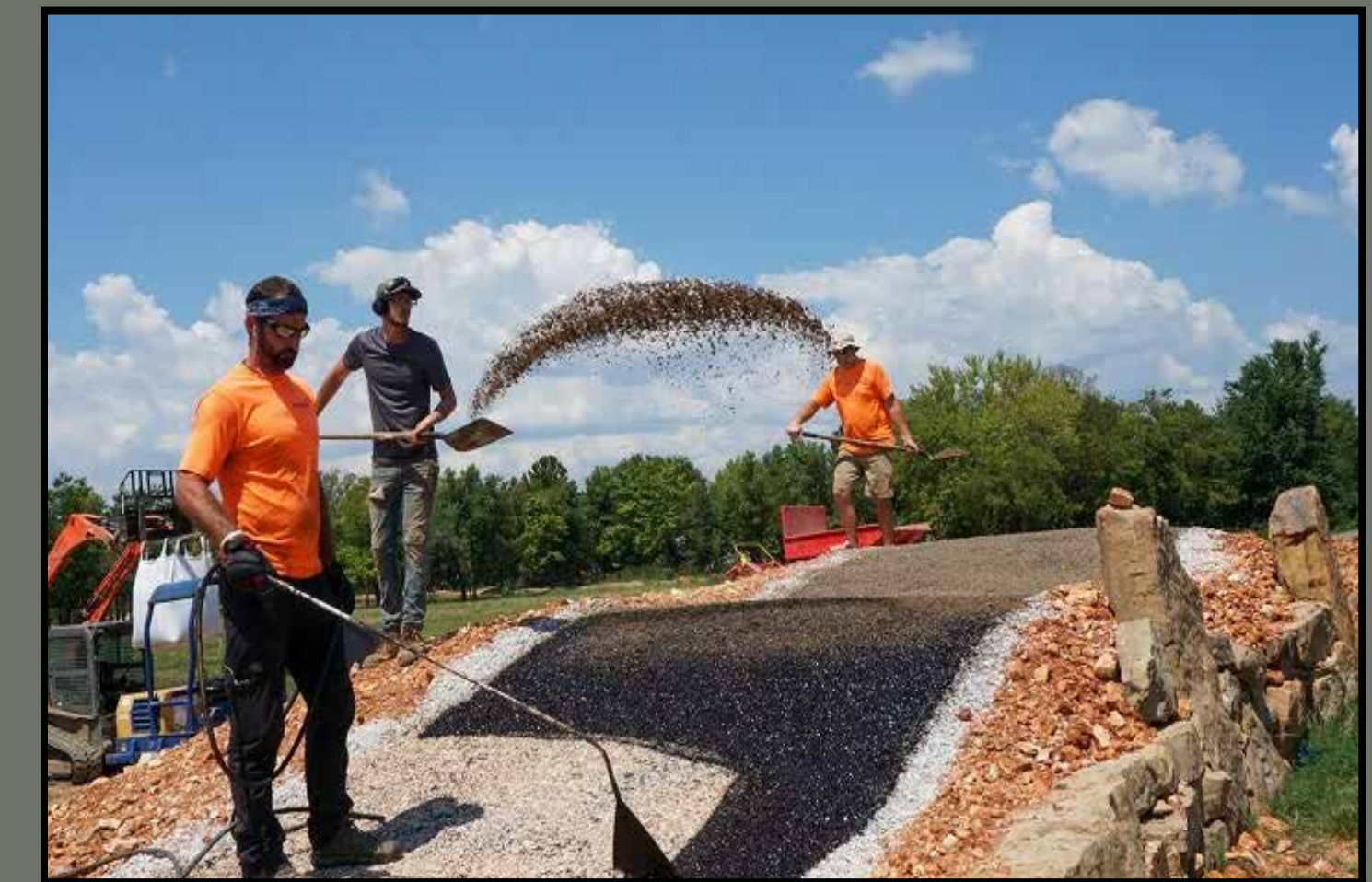
NO MAINTNENCE CHIP SEAL SURFACING
