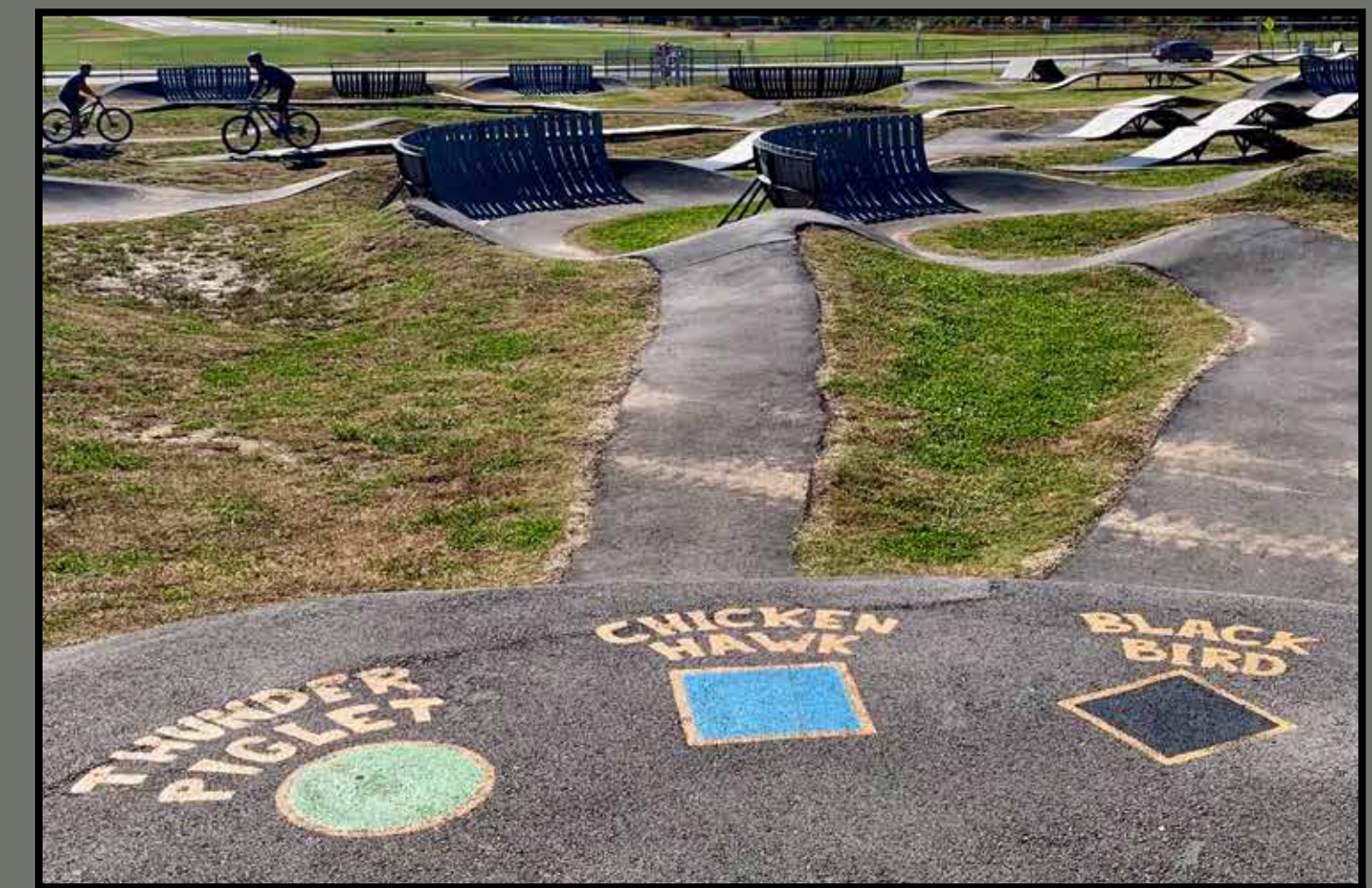
SLOPESTYLE ZONE - ASPHALT SURFACING
