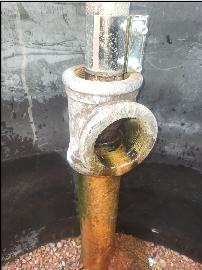
The artesian well at West End sprung a leak and the repairs have not fixed the problem.
