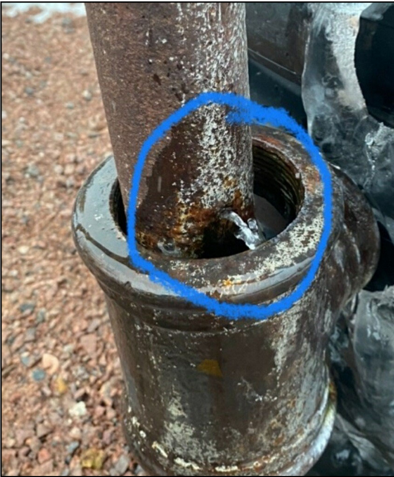
The artesian well at West End sprung a leak and the repairs have not fixed the problem.
